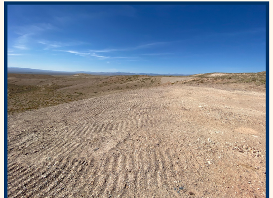
Additional cover material placed over previously reclaimed areas of the mine site having exposed acid generating rock, Nye Co., Aug. 2023.
